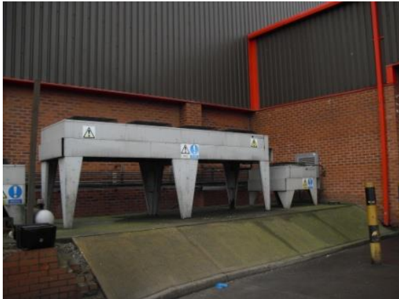
Photos taken from Pinneys DX R22 Freezer Plant with Air Cooled Condenser
