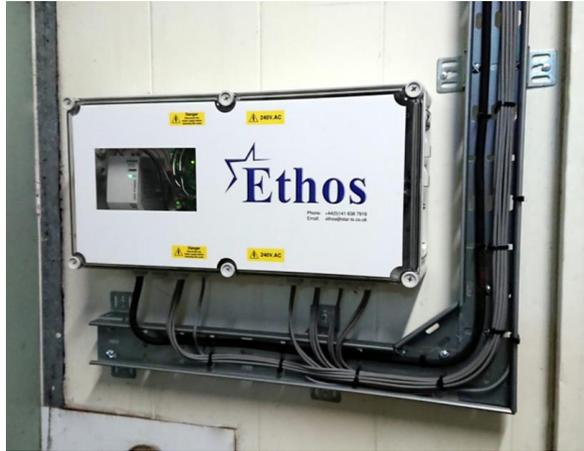
A standalone datalogger and set of sensors is installed
