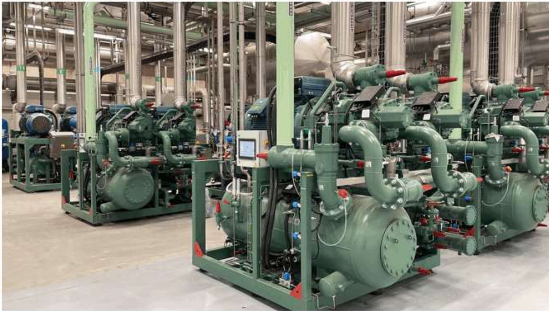
Dairy - Denmark 6 x ACP95103K-2C Q_o=12.000 \text{ kW} ; t_o=-0,5^\circ\text{C} ; t_c+30^\circ\text{C}
