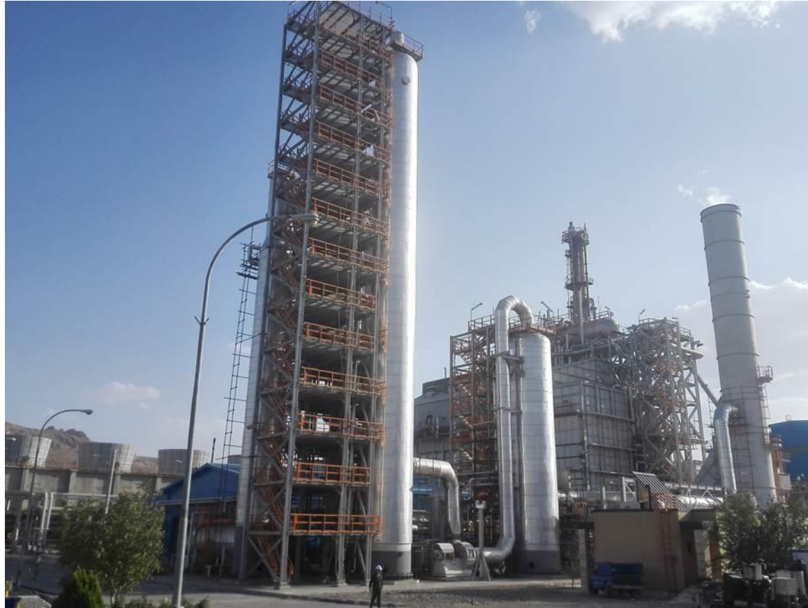
CO 2 from reformer chimney, Kermanshah Petrochemical
